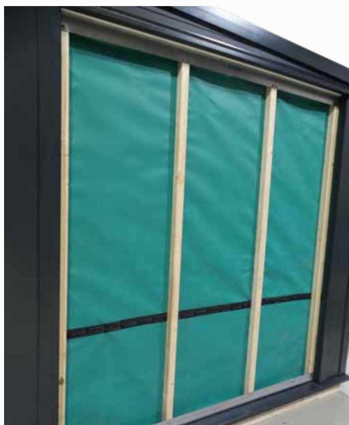
Wall prepared for cladding - battens supplied
